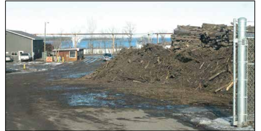
Stockpiled railroad ties provide fuel for the L'Anse Warden biomass facility.
