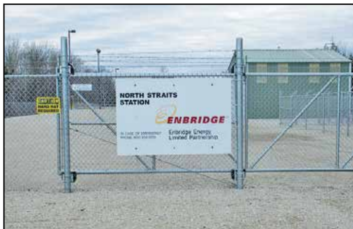
Pumping and control station for Enbridge Pipeline 5 on the Upper Peninsula side of the Mackinac Straits.
