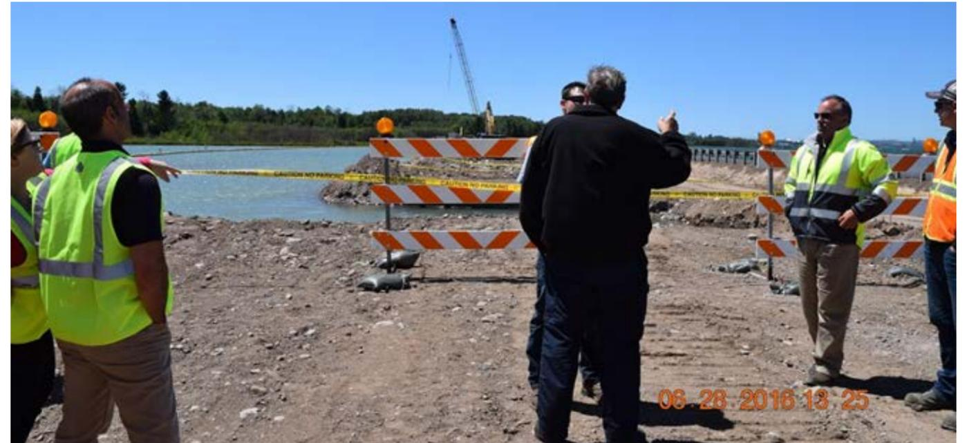
Bridge construction on St. Mary's Rapids with SPAC group tour. The bridge pad is behind safety sign. A portion of the old causeway on the right will be removed.
