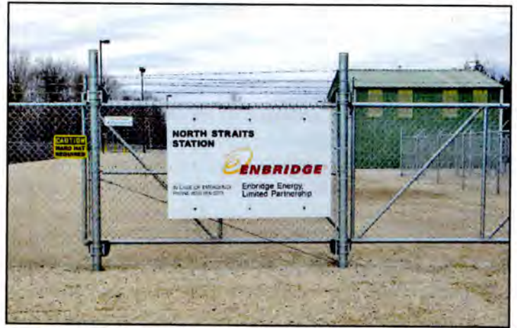
Pumping and control station for Enbridge Pipeline 5 on the Upper Peninsula side of the Mackinac Straits.
