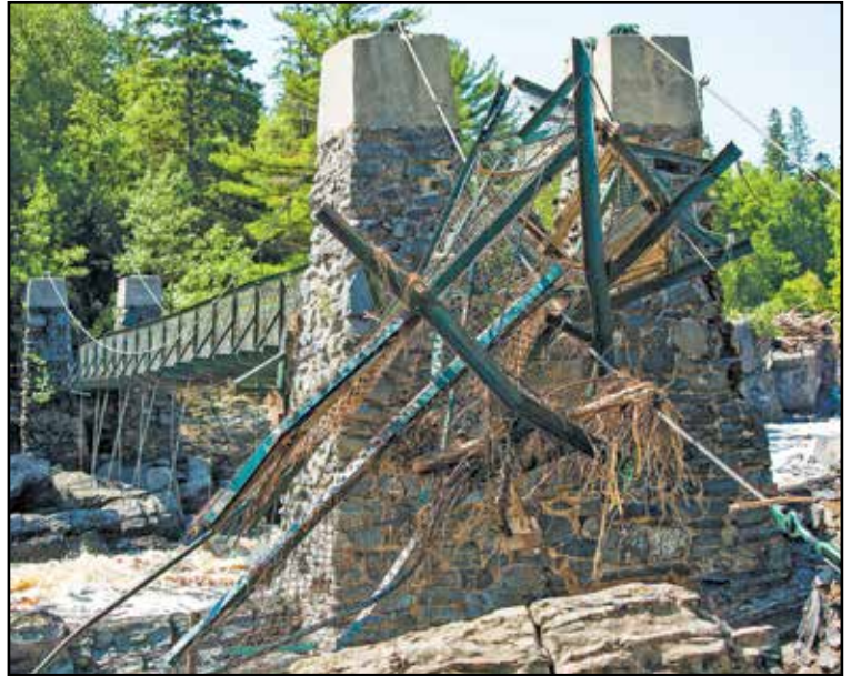
The swinging bridge at Jay Cooke State Park devastated by a record-high St. Louis River (above). Below is one of many mudslides along Chester Creek that resulted in fall line trails being wiped out. See more of Derek Montgomery's work at derekmontgomery.com
