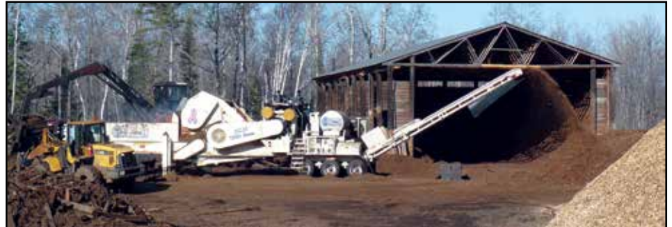
A railroad tie chipper operates at the L'Anse Warden electric power plant. In 2014, Michigan Legislature's redefined railroad ties and tires as biomass and renewable, thus legal as combustion additives.
