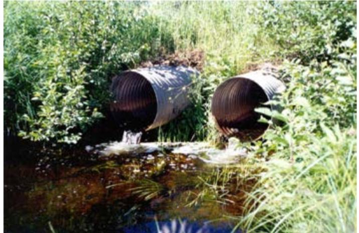
The worst possible stream crossing is a “perched” culvert (above.) Fish would have to jump to enter the downstream end of this culvert and then make its way with high velocity over the steel corrugation which is normally impossible. There are numerous examples of perched culverts around the Western UP where I managed trout for the DNR during my career. Many other culverts are undersized and block trout with flow velocity or placement that is too much for trout to swim upstream through them.
